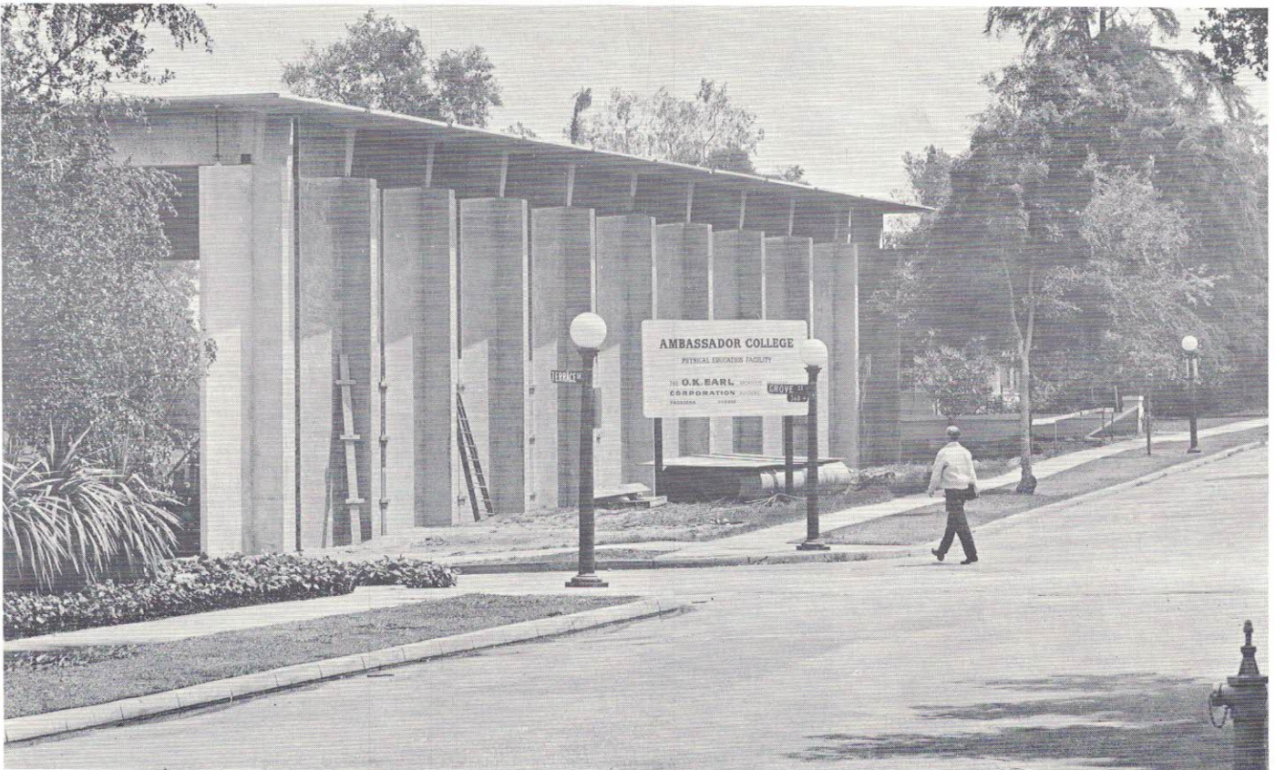
A first for Ambassador! Unique construction sets precedent for rest of world! Completion date is August.
